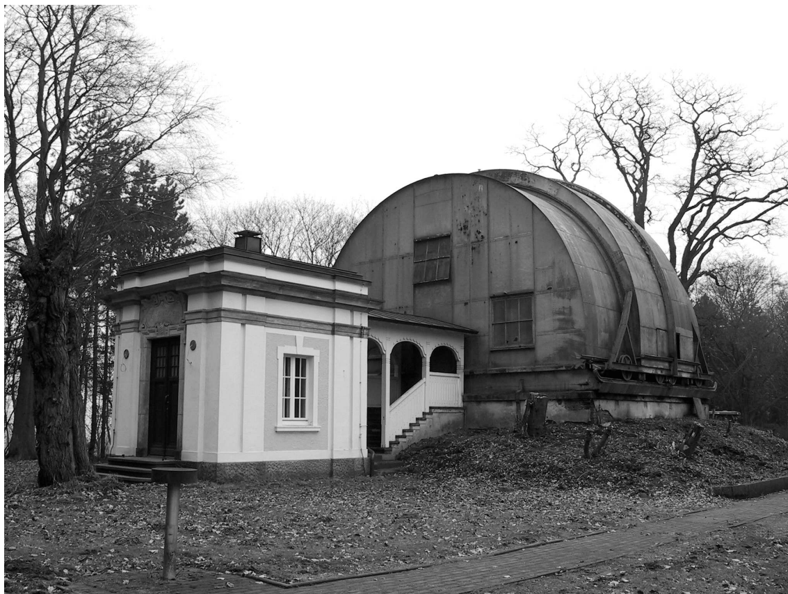
Figure 7.2: Meridian circle building
